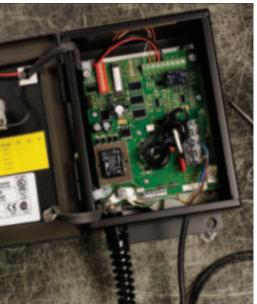
With TraceCheck<sup>™</sup>, a feature of the controllers, you can be sure your heat tracing is working when you need it because the feature exercises dormant lines every 24 hours for early warning for shutdown prevention.
